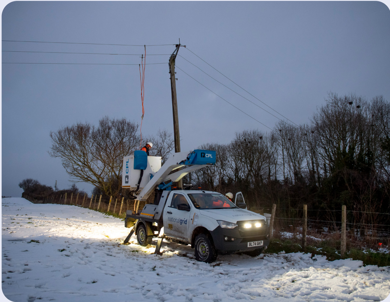
Colleagues working on overhead lines during Storm Goretti.
