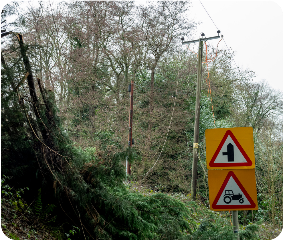
An overhead line brought down by a tree during Storm Goretti.
